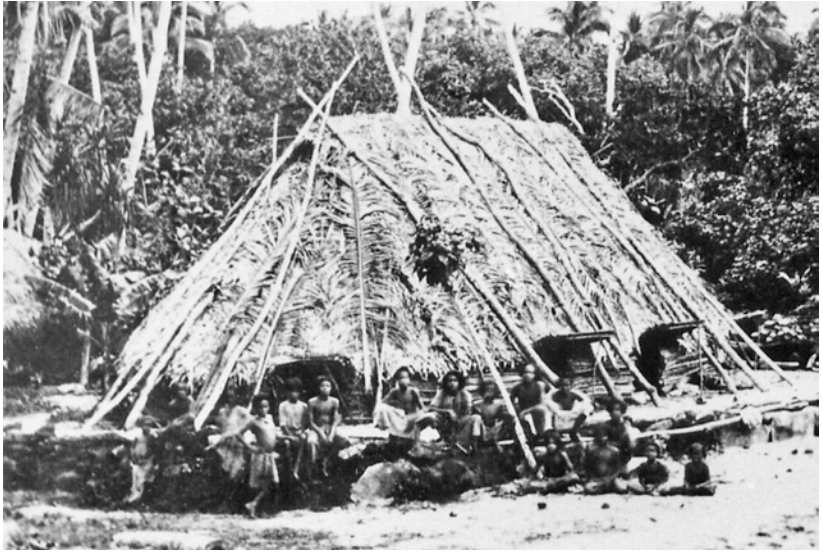
Photo 2.4 Traditional Rotuman house. Note raised-earth foundation with stone walls. © Fiji Museum.
