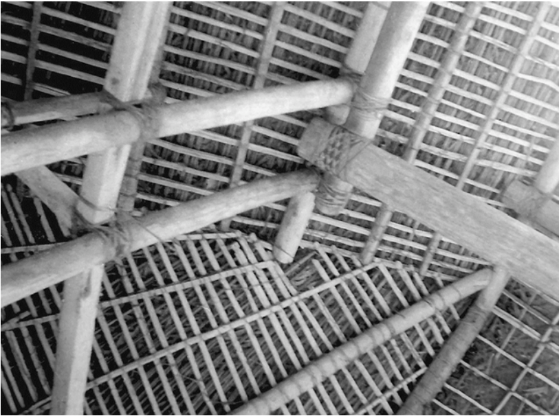
Photo 4.16 Detail of timbers and roof at junction of side and curved end, 1940. H. S. Evans.
