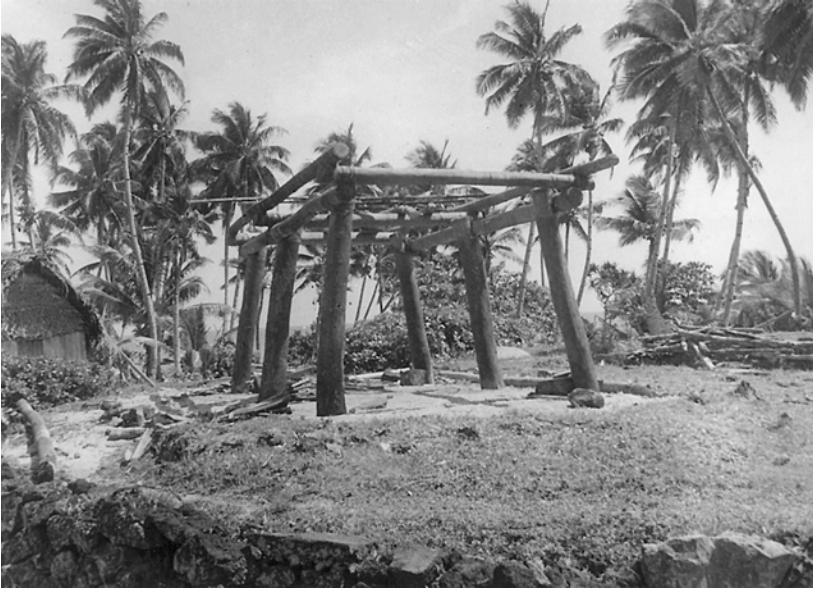
Photo 4.15 House building with double-sided top plate, 1940. H. S. Evans.
