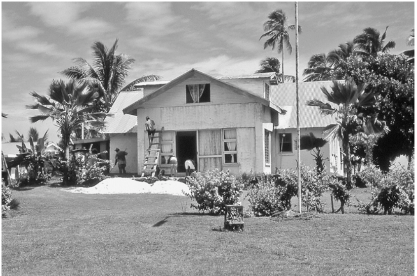
Photo 12.11 Men painting a modern, two-story home, 1989. Jan Rensel.
