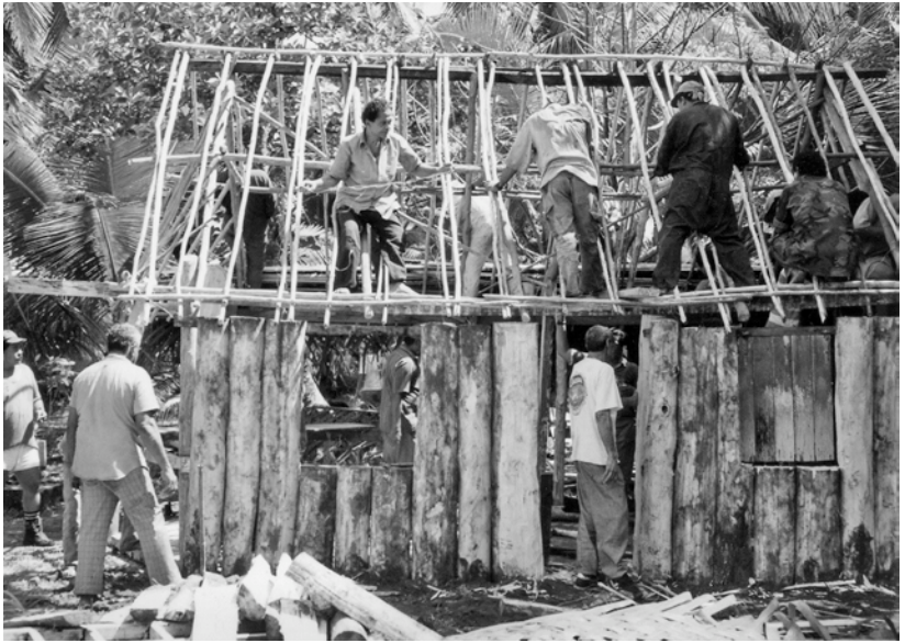
Photo 12.10 Men constructing a thatched-roof house with timber walls, 1989. Alan Howard.
